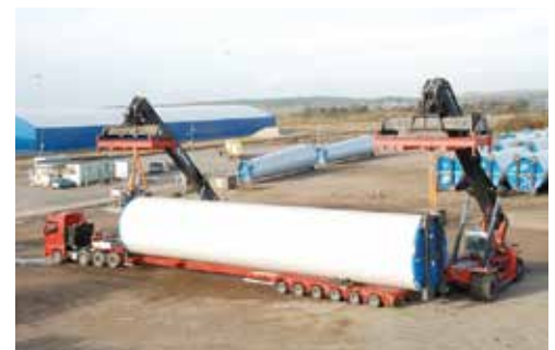
Off loading of truck at storage area.
