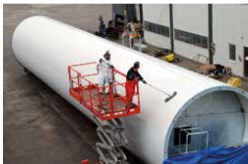
Cleaning of tower sections
